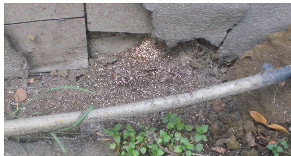
Vermiculite shown leaking from siding on the exterior of a structure
